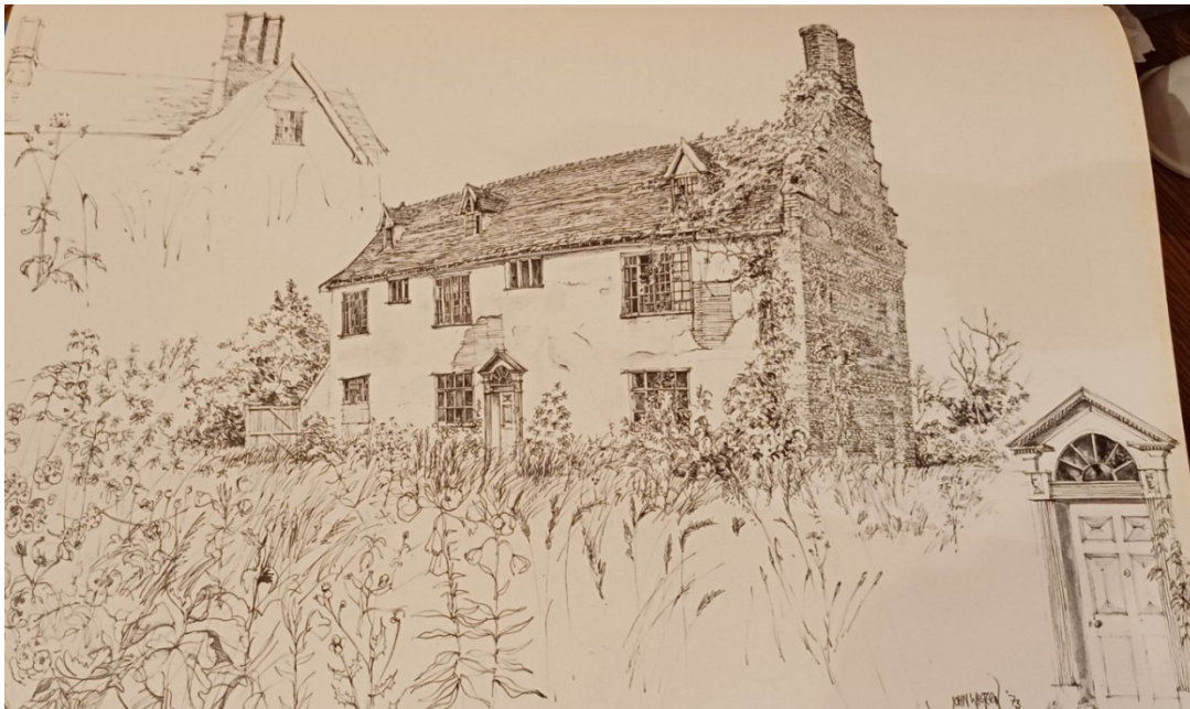
“Hempnalls Hall, Cotton. View from the West prior to Restoration” xx 1977
