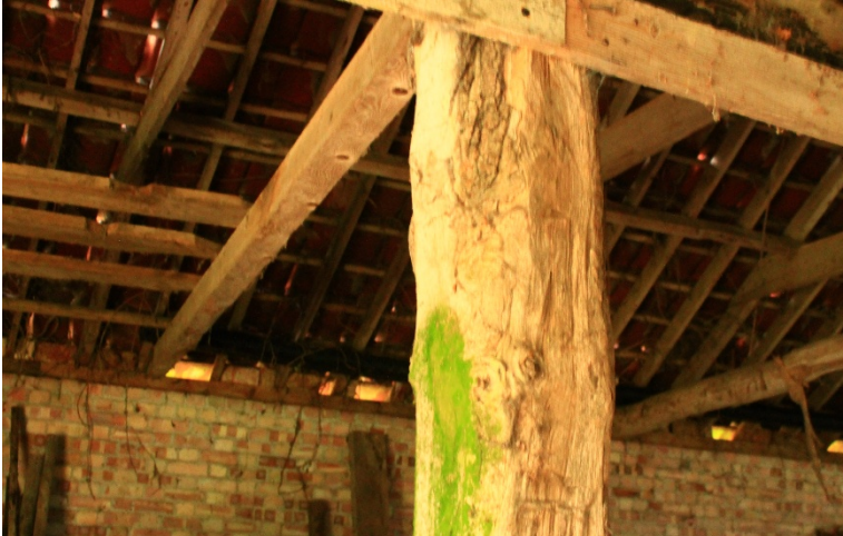
One of a row of evenly spaced beams - possible former stables
