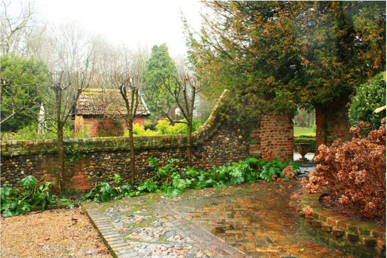
Arch to topiary garden with bricked up arch to the left, mature yew to the right Some constructions sit upon older sections of wall of unknown age, such as that shown below.
