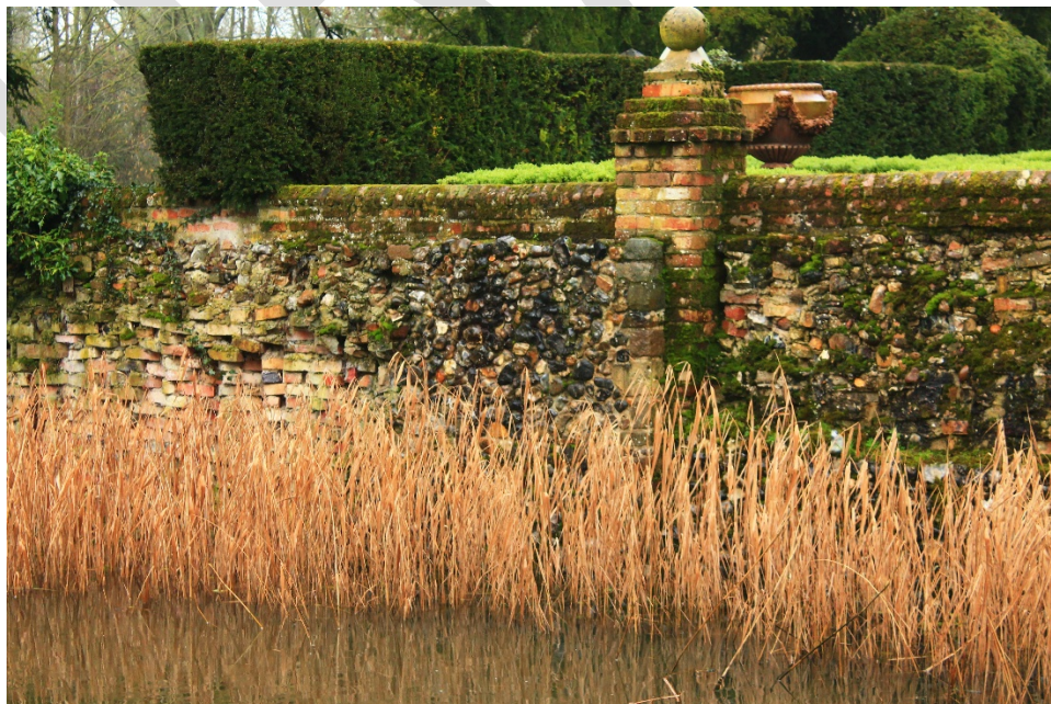
Revetment, wall and post, fronting moat
